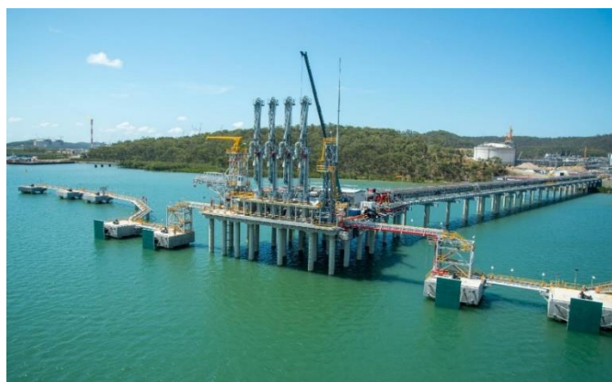
Figure 3-7 An Example of the Jetty
