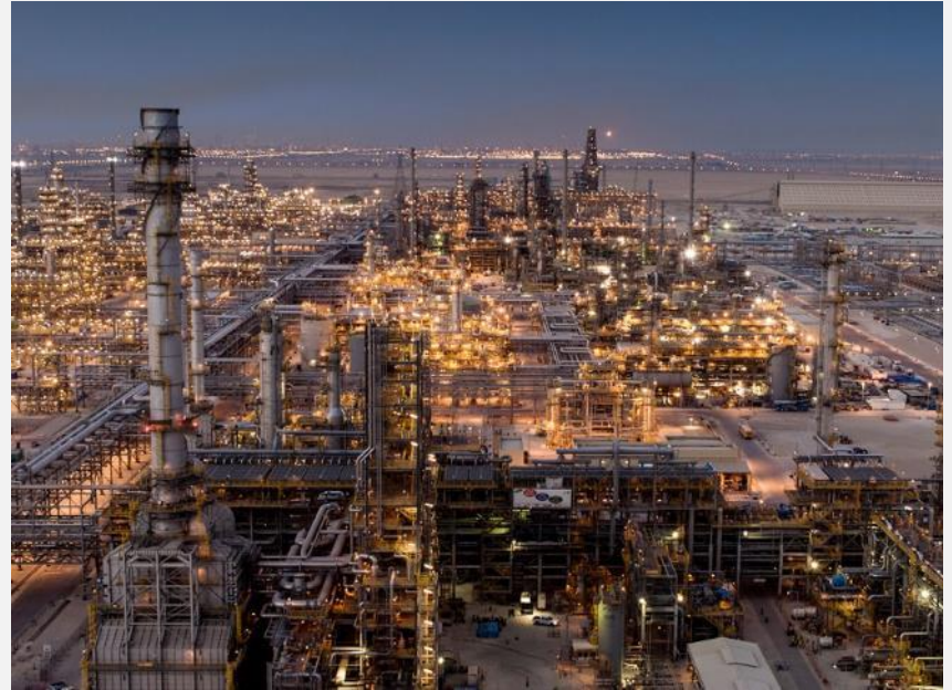
Satorp refinery, Saudi Arabia
