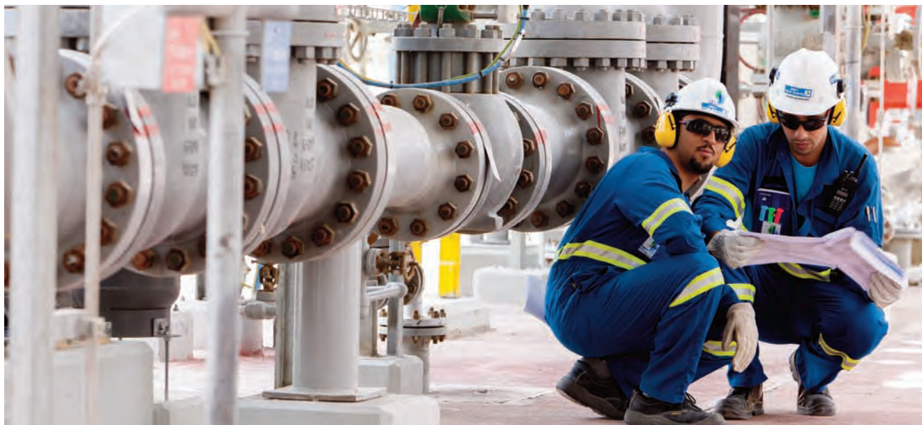
Outside operators at the Satorp refinery in Jubail, Saudi Arabia
